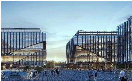
a double glazed curtain wall, where both elements work together to reduce the thermal transfer through the building. The form of the building and the design of its facade have been proportioned to provide natural day light through an optimum organization of office space to encourage a healthier and productive environment.
