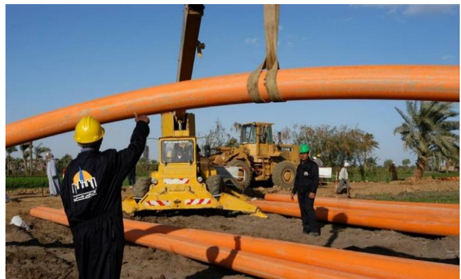
TAQA Gas Pipe-Laying Works
