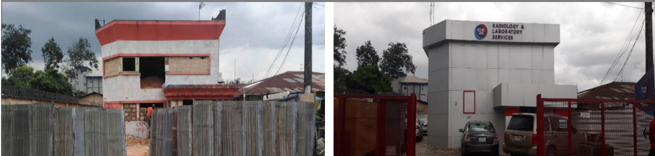
Benin Branch Renovation & Rebranding
