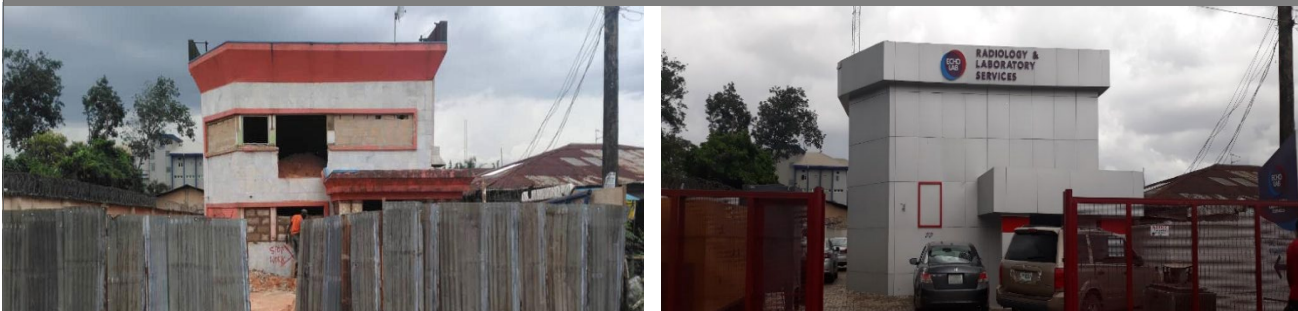
Benin Branch Renovation & Rebranding
